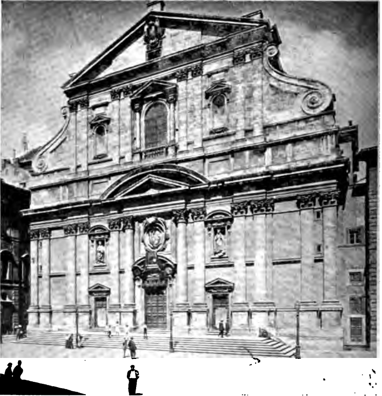
FAÇADE Church of the Gesù, Rome
